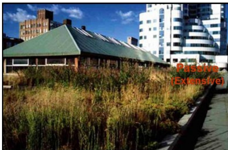
Figura 04- Cobertura extensiva – Fonte: City of Toronto – What is a Green Roof – www.toronto.com
